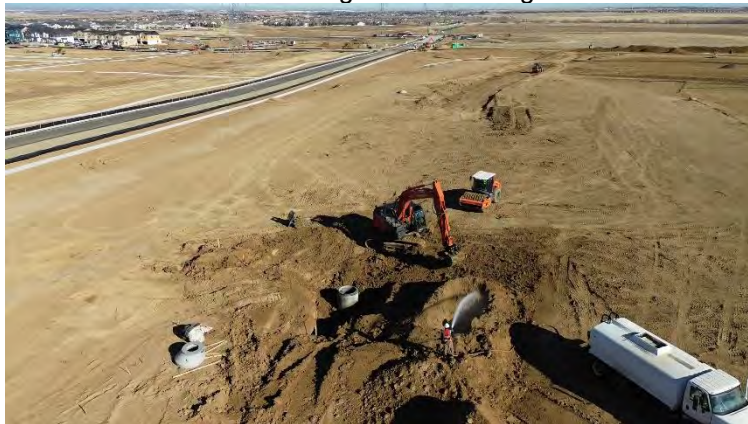
South Portion of Site – Facing Northwest
