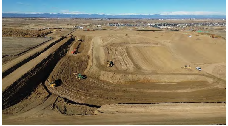
Filing 1 Overall View – Facing West
