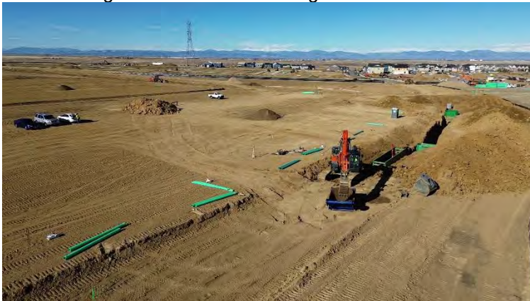
Sanitary Sewer Installation – Facing Southwest
