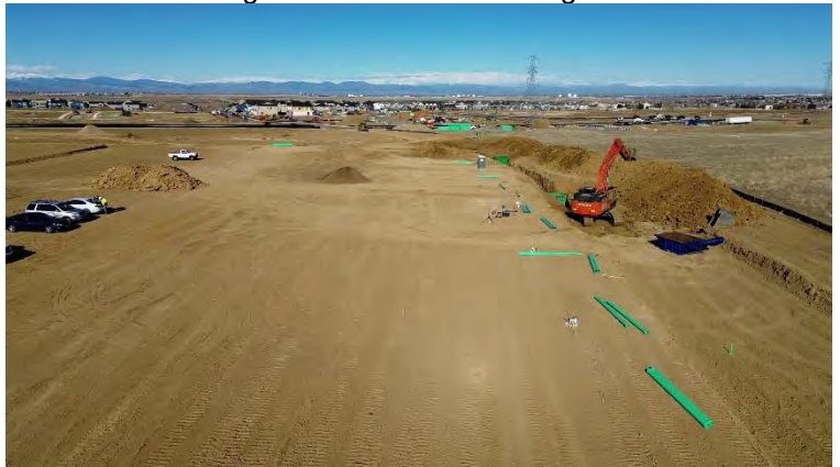
Sanitary Sewer Installation – Facing West
